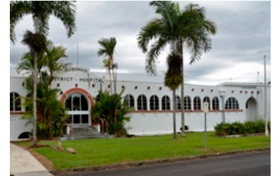
Mossman District Hospital, May 2013. Image NTQ files.
